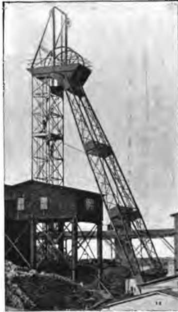
FIG. 529.—Pit-frame, lattice girder (Mansfeld).
